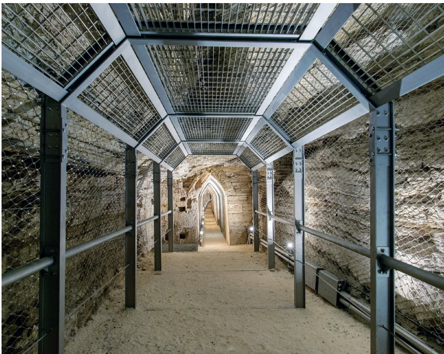
Fig. 20. The protective canopy between the Archaic and the Roman lining, view from north (Ch. 49–63.9)
