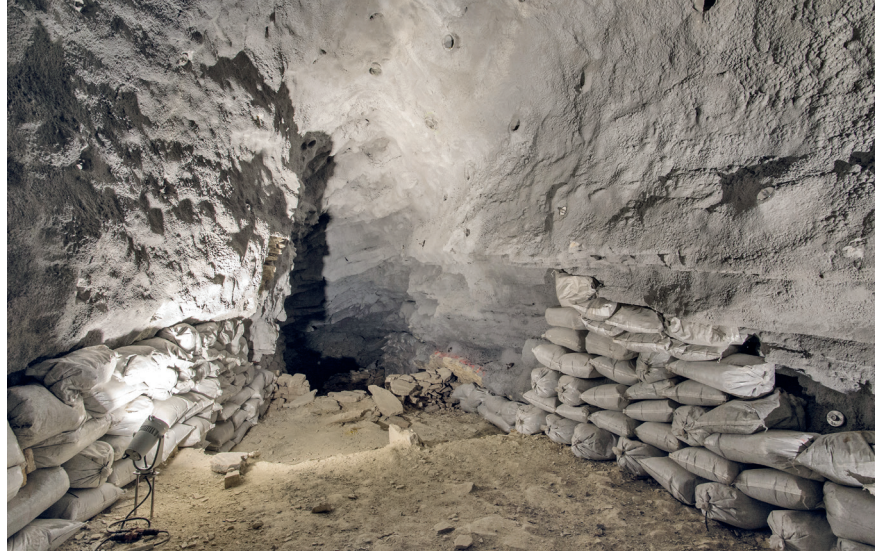
Fig. 21. The cave above the Roman lining protected by anchors and shotcrete
