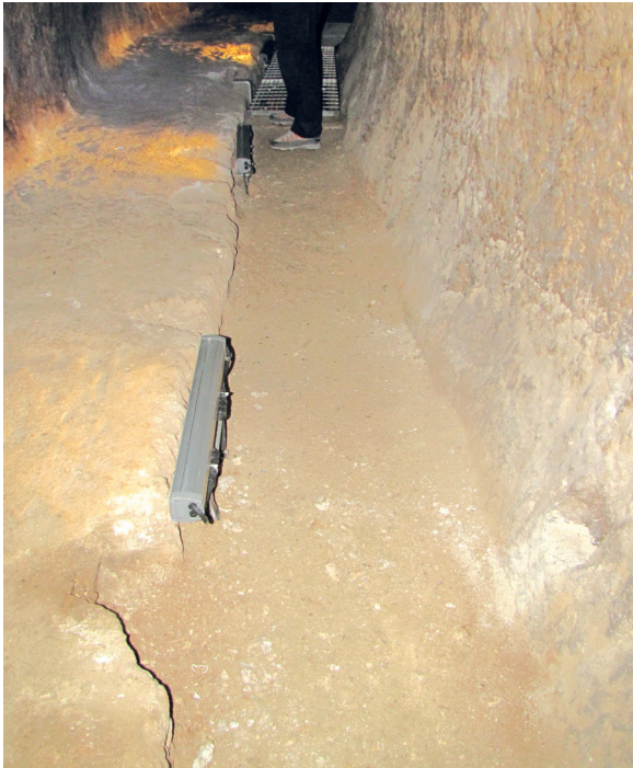
Fig. 31. Notches on the edge of the floor and on the wall above a bridge between Ch. 765 and Ch. 770
