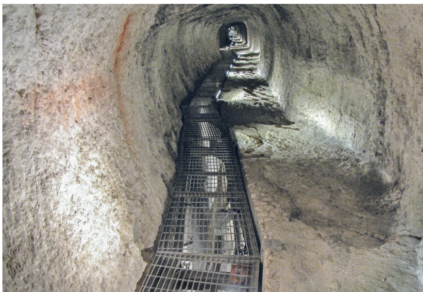
Fig. 24. The tunnel with the steel gratings and the new illumination with LED lights, view from the north (from Ch. 855, before the inscription ΑΡΙΣΤΕΙΑΩ)
