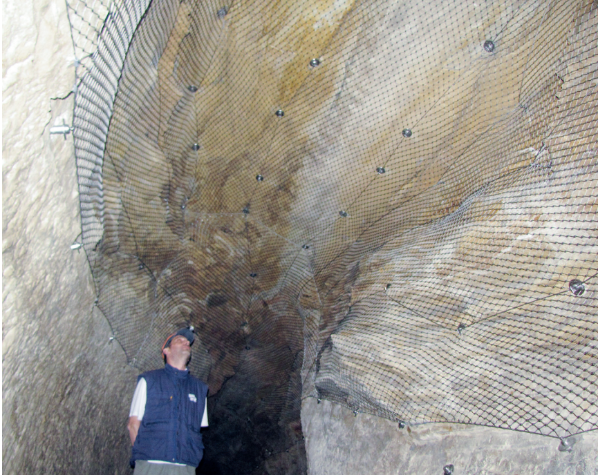
Fig. 19. The wire net with the anchors (Ch. 660)
