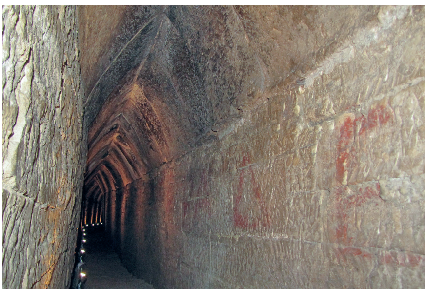
Fig. 25. The Archaic lining with the new illumination with LED spotlights, view from the north (from Ch. 174)
