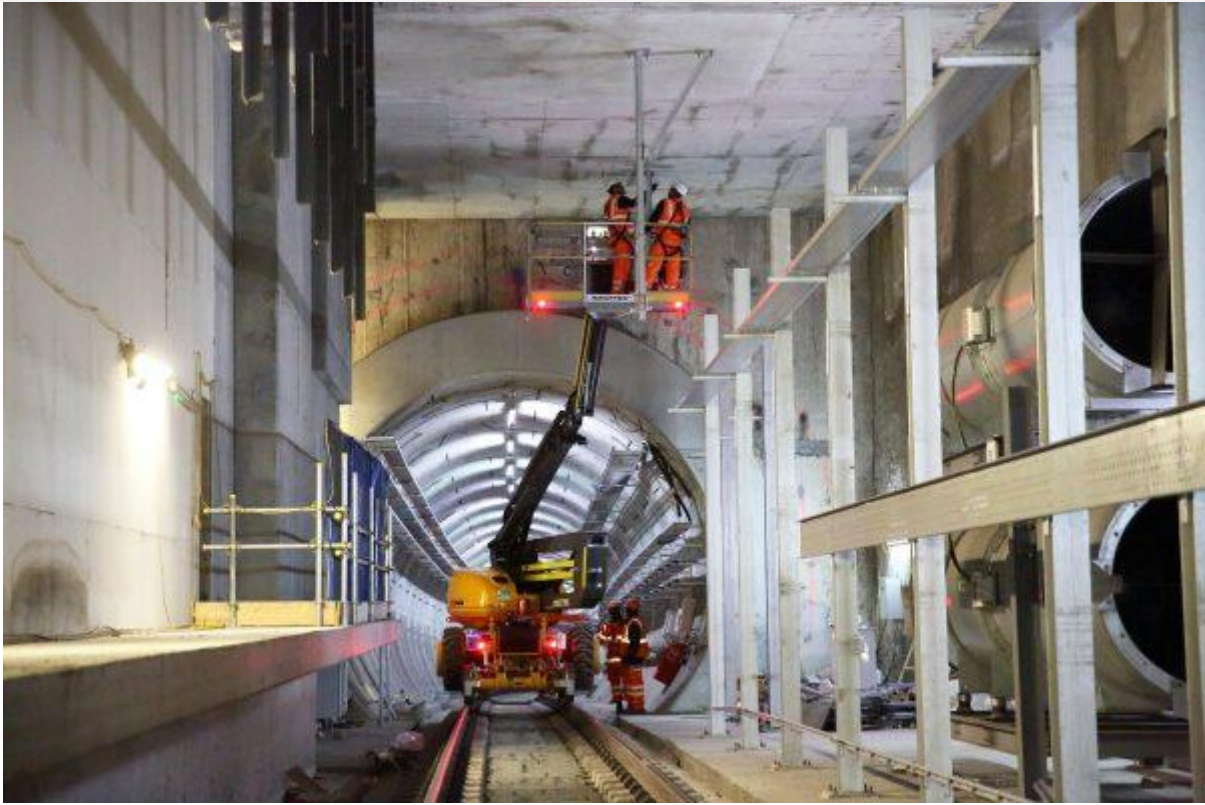
Installing overhead catenary system in the Thames Tunnel_246115
