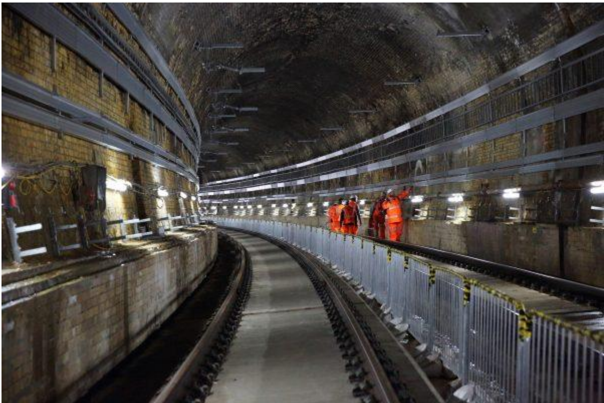
Installing overhead catenary system in the Connaught Tunnel_266105
