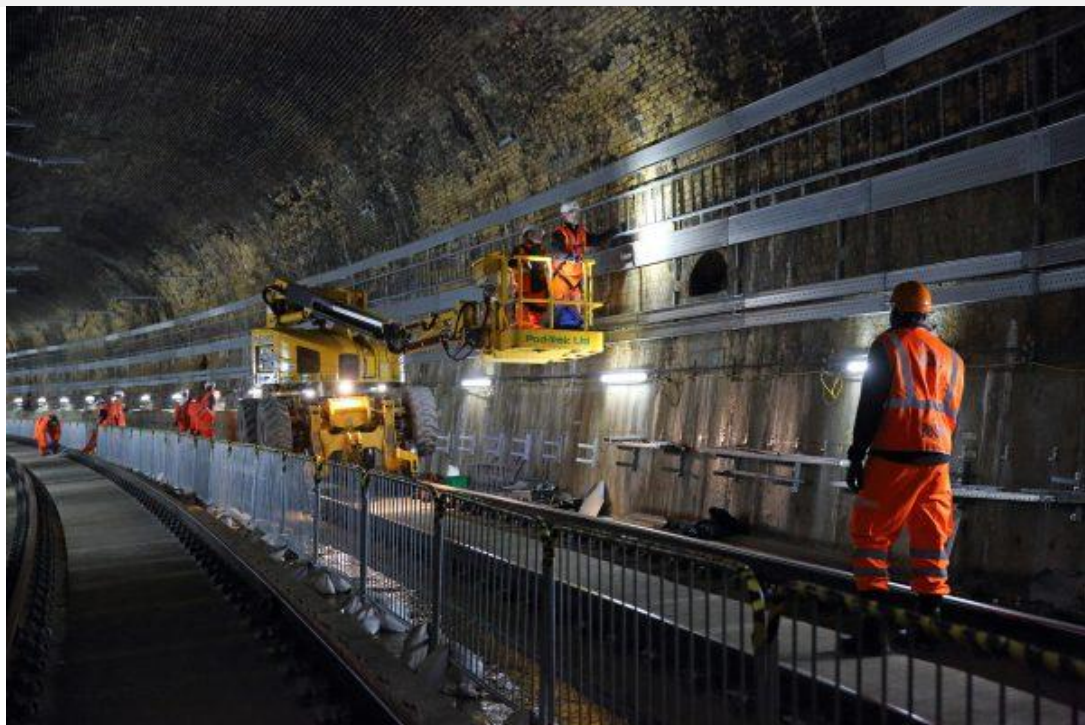
Installing overhead catenary system in the Connaught Tunnel_266101
