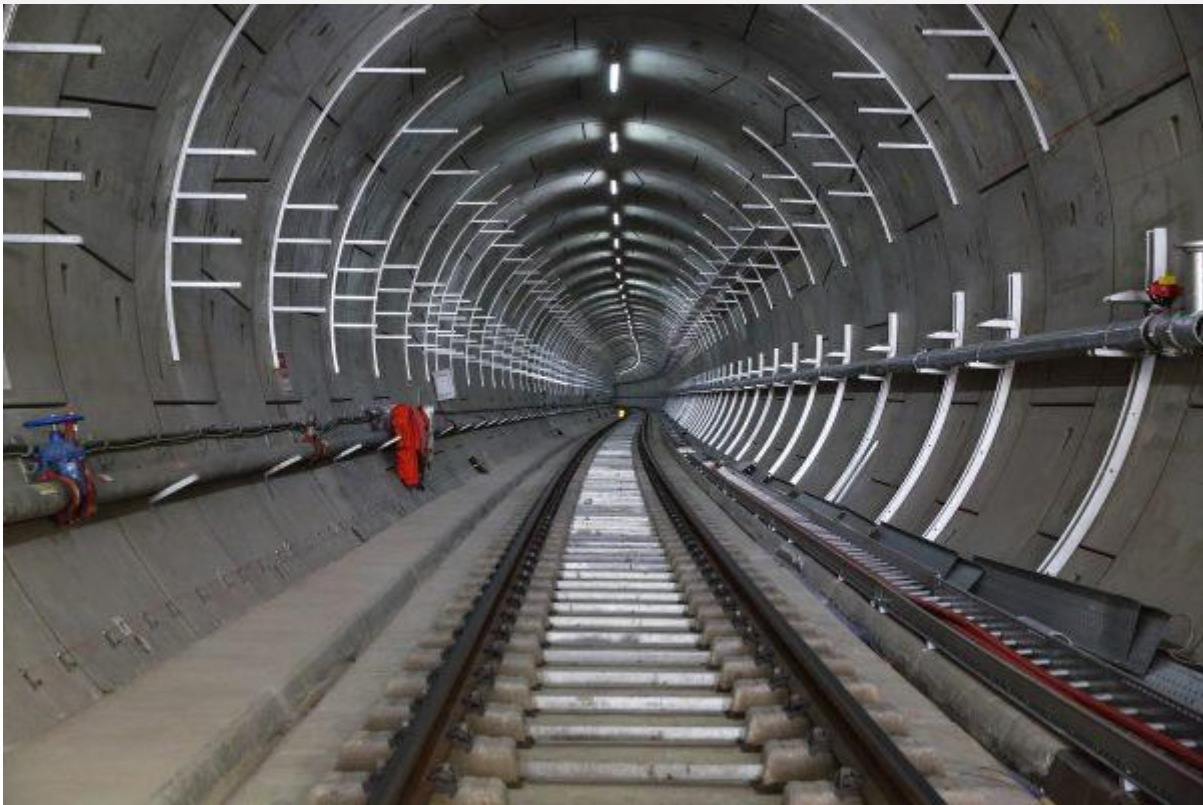
Cable management Cable management systems installed in Crossrail tunnel_268041
