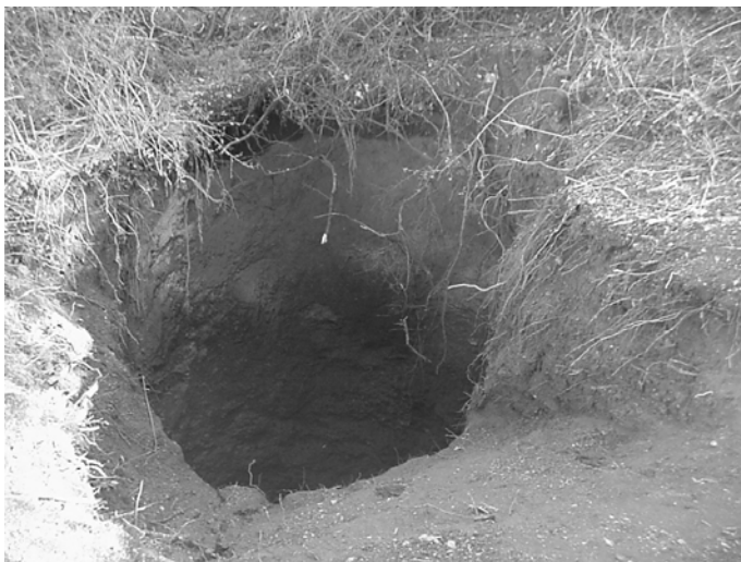
Figure 8: Collapse of the filling of a karstic chimney crossed by Dodoni Tunnel. The collapse outcropped on the surface about 100 m over the tunnel
