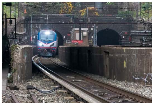
(Photo: Tunnelling Journal)
