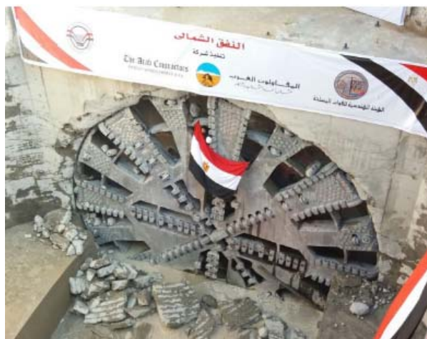
(Photo: Tunnelling Journal)
